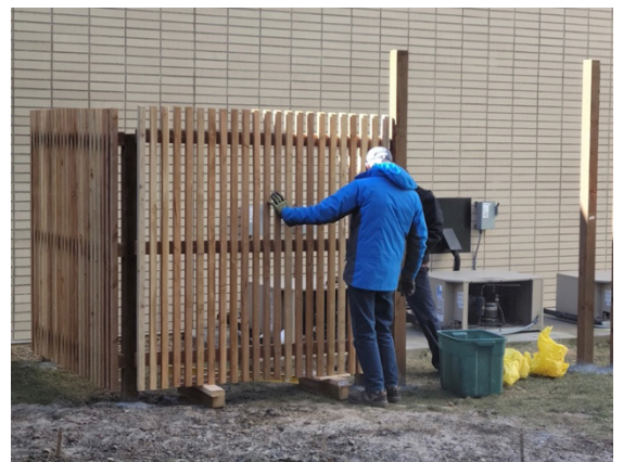
Outdoor Campus Committee Chair Cliff Hillebrandt constructs the trellis screen for the new garden.
