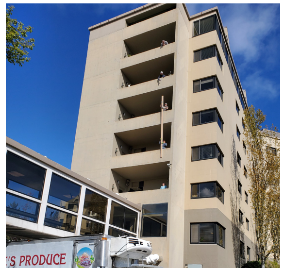
Where there's a will, there's a way! Construction workers hoist beam to upper floor. Photo by Walt Lundberg
