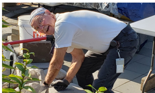
Left: Robin Bolton is laying the tiles in the new Tower Garden Patio. See story on page 9.
