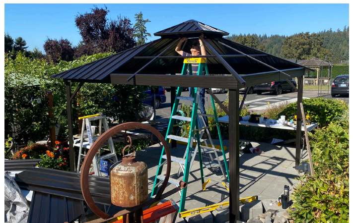
Cliff Hillebrandt completes roof installation on the new pergola in the Tower Garden Patio. Details on page 9.
