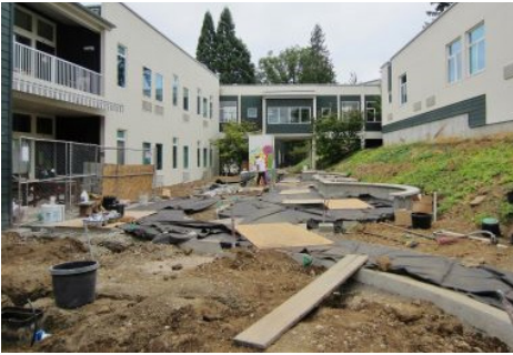
Harmony Garden construction – 2012
