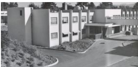
WV Hospital Phase 2 addition – 1959; currently it is the Plaza building. South wing is on far right past the skybridge.
